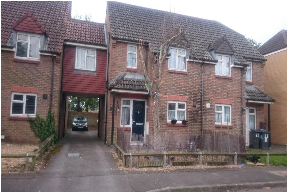
BH10 7HY - 24 Keeble Crescent
