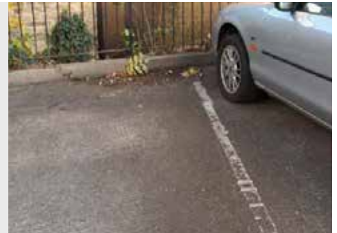
Grade B - Satisfactory
