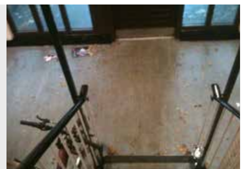
Grade D - Very poor
