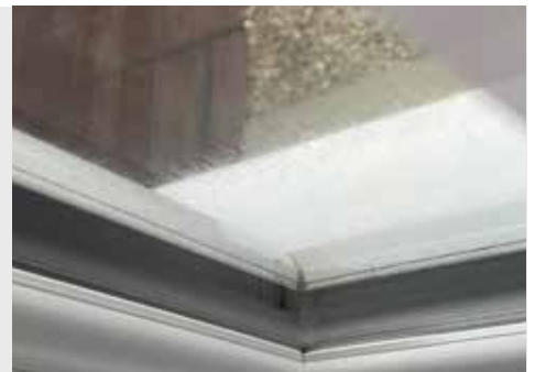
Grade B - Satisfactory
