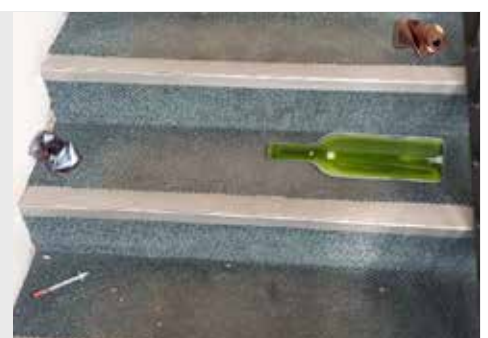
Grade D - Very poor
