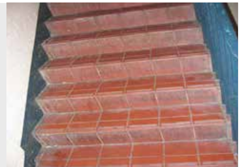
Grade B - Satisfactory
