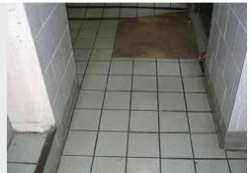
Grade B - Satisfactory
