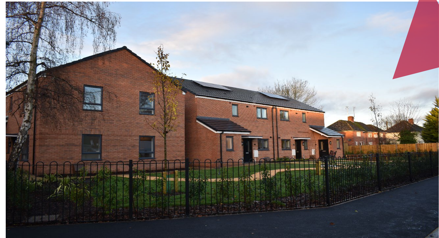
Waterworks Lane, Leominster Veterans' self-build
