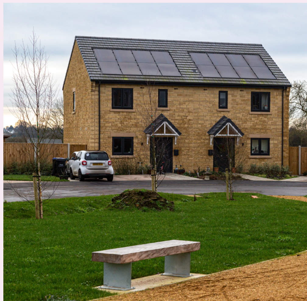
Our Station Road, Holt, Wiltshire, development.
